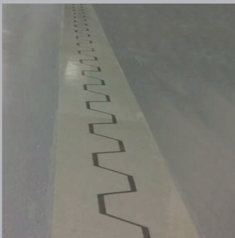
Smart Joint ® applied on finished resin floor
