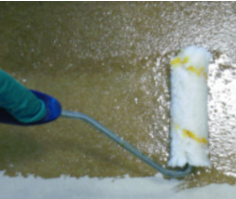
Application of Mapefloor I 910 as adhesion promoter
