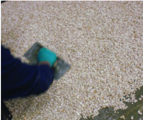
Application of the Mapefloor I 910/natural aggregates mixture
