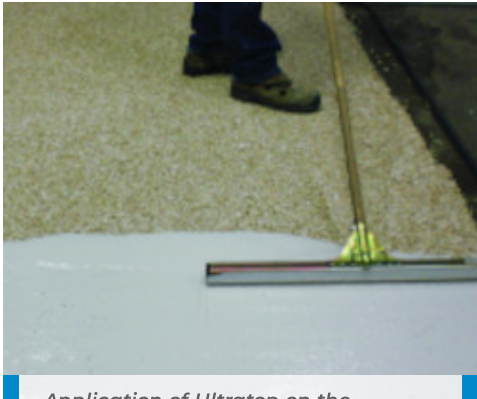
Application of Ultratop on the hardened surface of the Mapefloor 910/natural aggregates mixture
